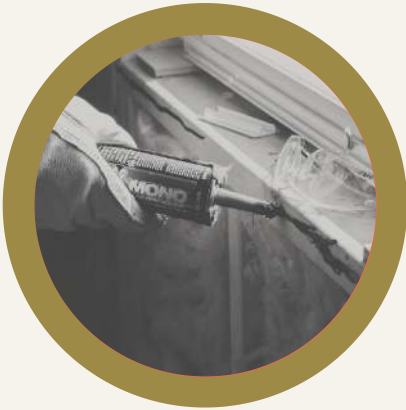
Renovation Works 25 Weeks of Trades onsite
